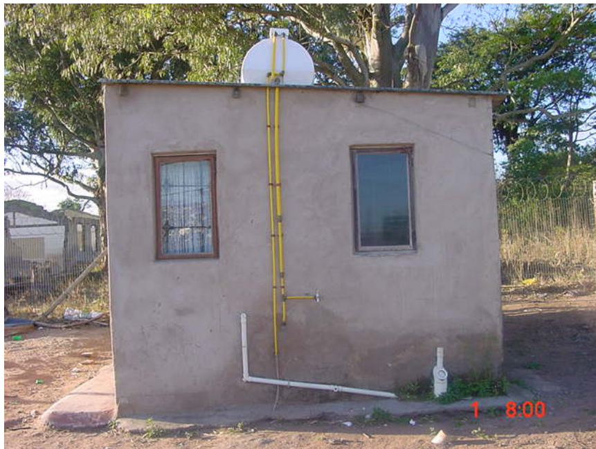
A roof tank in Durban, South Africa
